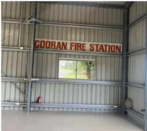
Cooran Fire Station, QLD Epoxy floor
