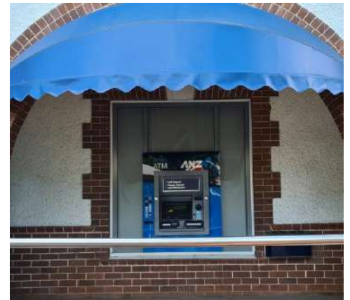
ANZ Casino, NSW Entry area
