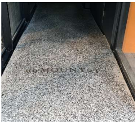
99 Mount Street Sydney, NSW Epoxy car park & Entry area
