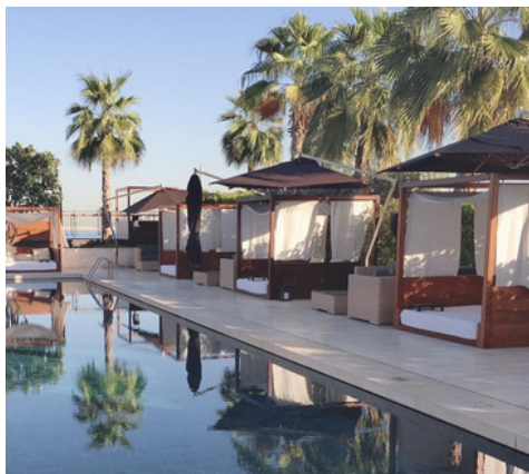
BULGARI Resort, Dubai Marble tiles, pool area: 250m2
